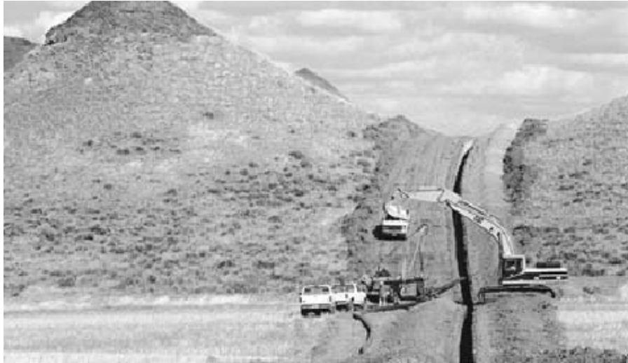
Figure 3; Trenching for transportation of product water at Yukon, Source; CPAWS-Yukon, 2008.
